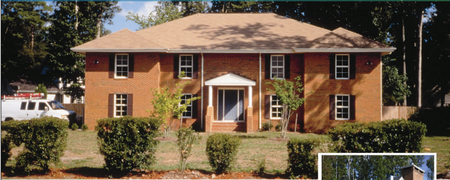
HRSD pump stations
